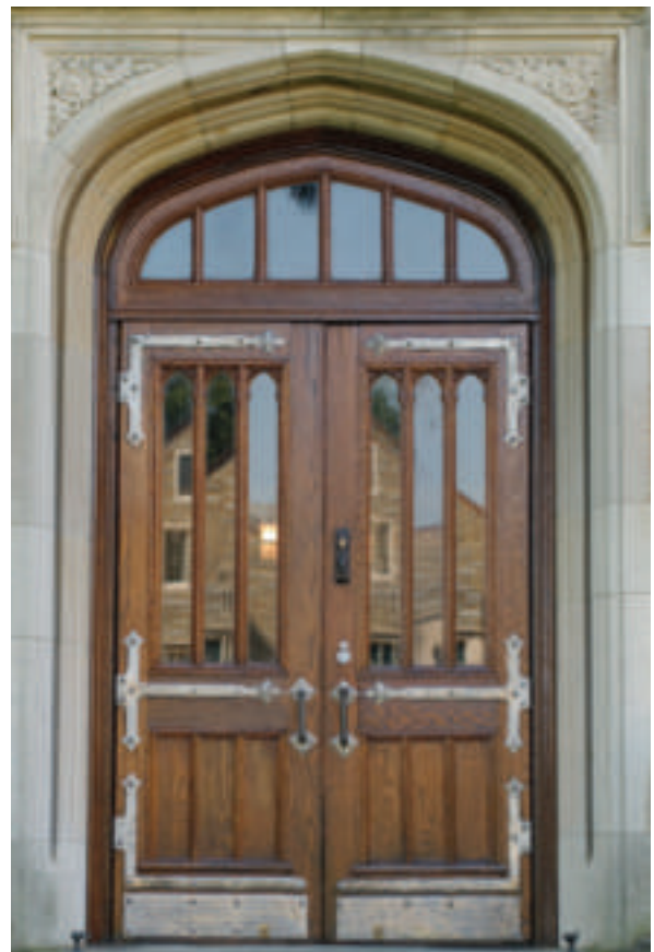
Following a summer restoration, the doors of Founders' Hall look just like they did in 1930.
